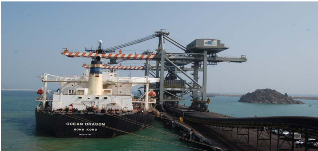
MV Ocean Dragon at Gangavaram Port Coal Berth
